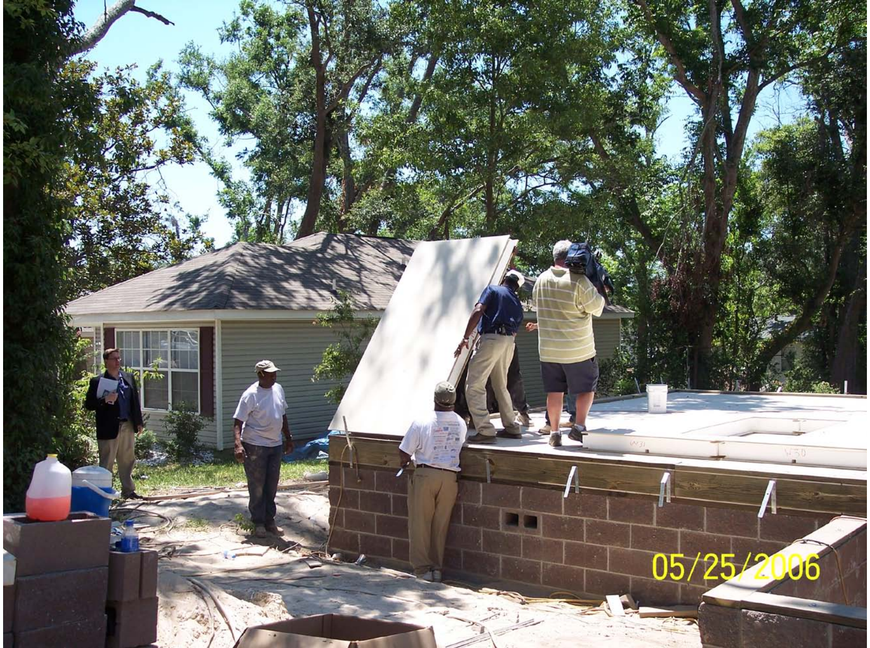
Installing the first exterior wall panel
