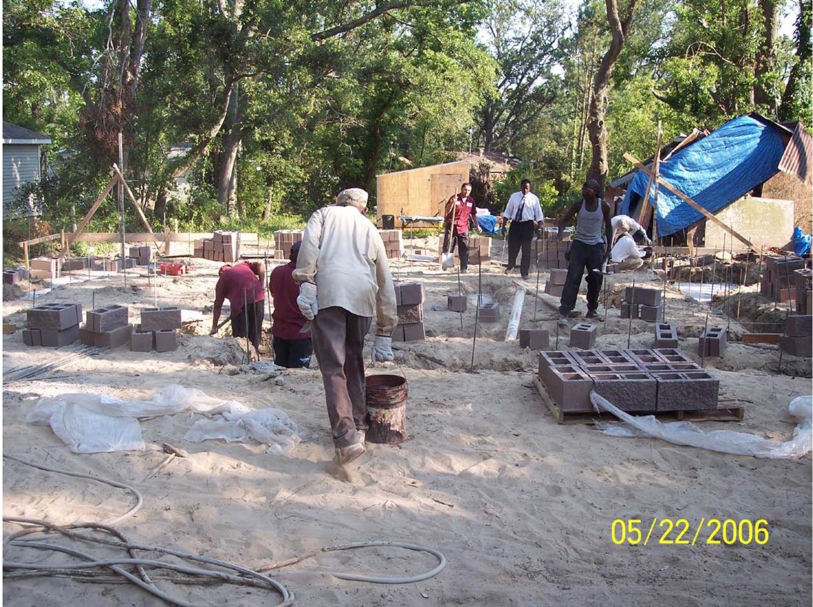
Laying the foundation
