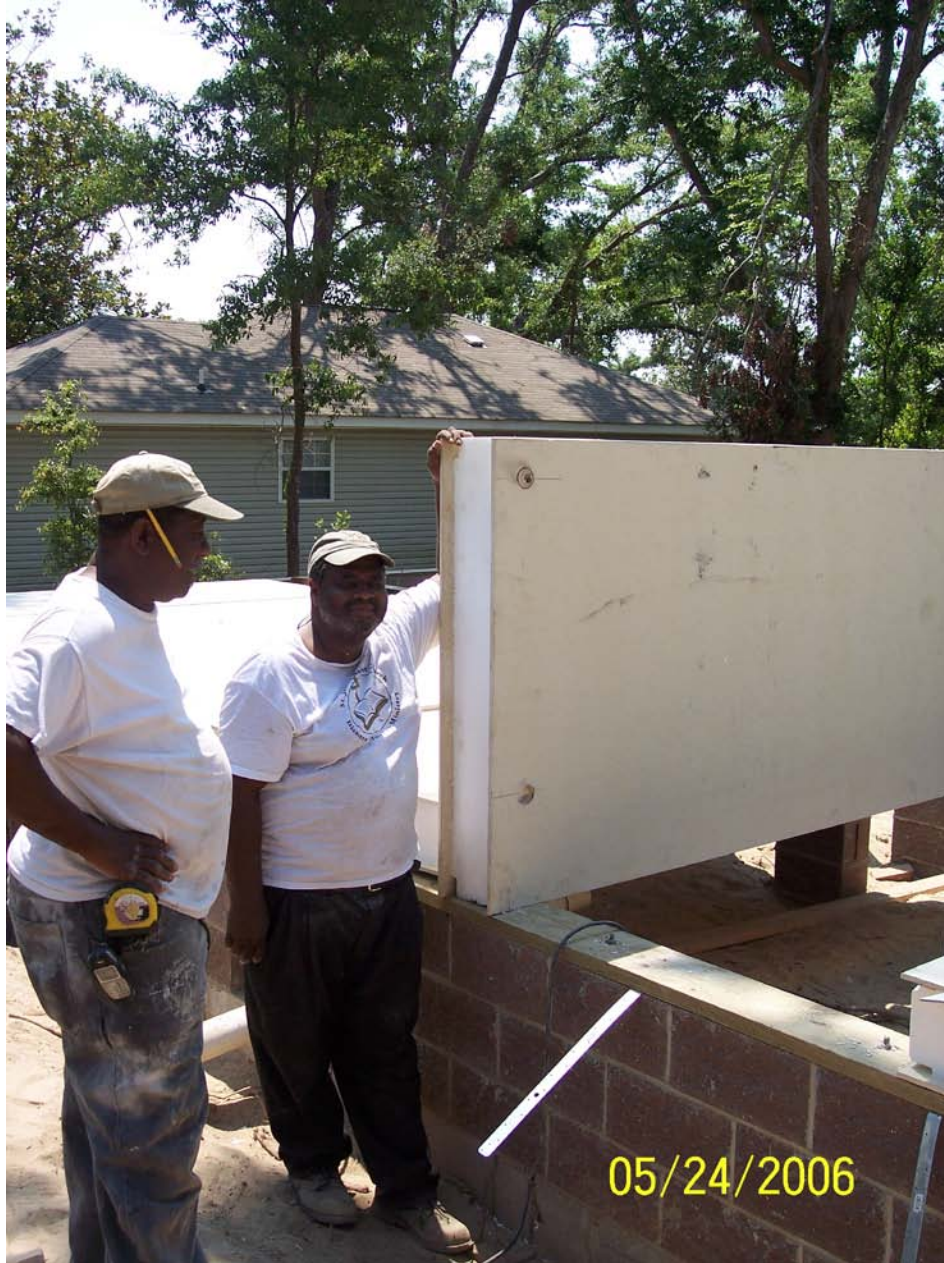
Preparing to lay the floor panels
