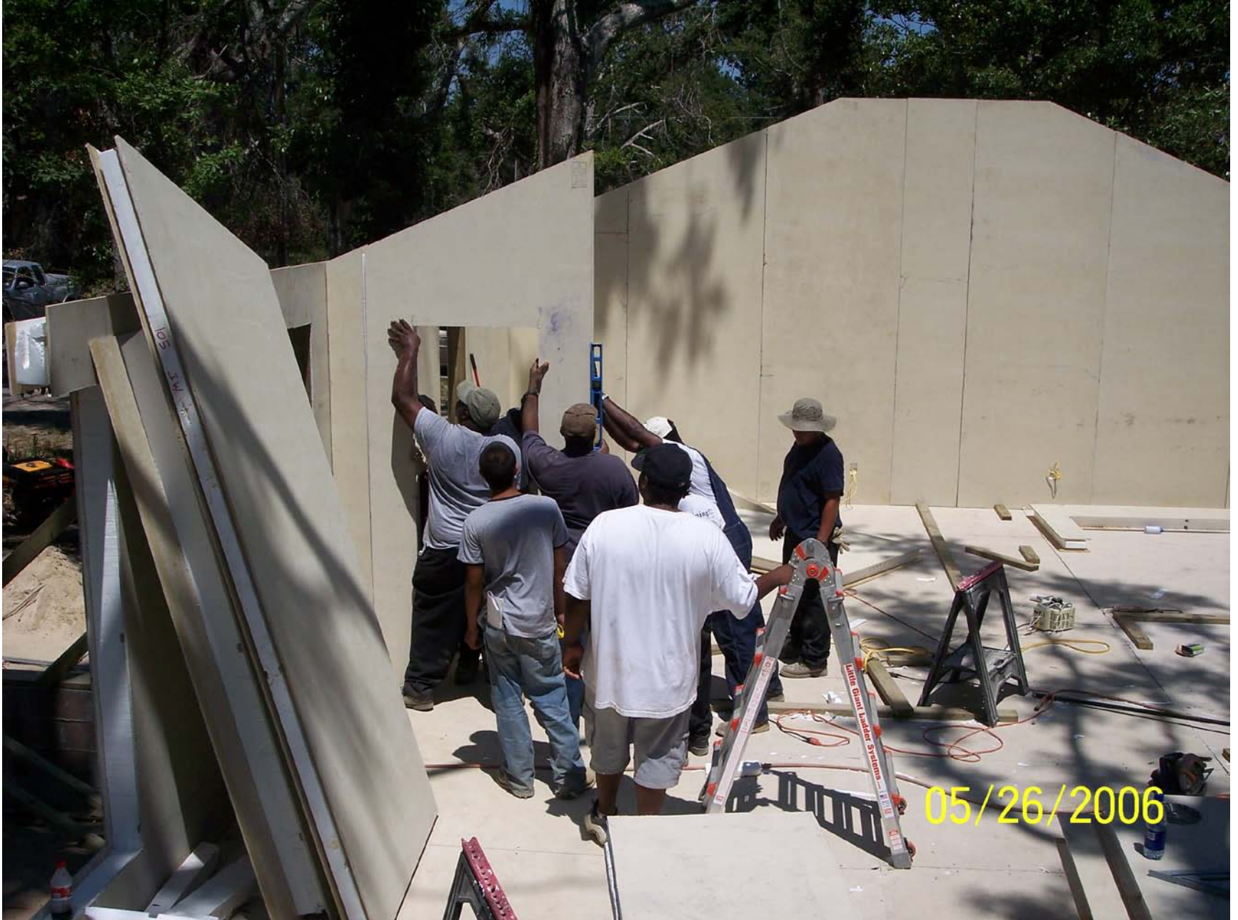
Erecting the interior walls
